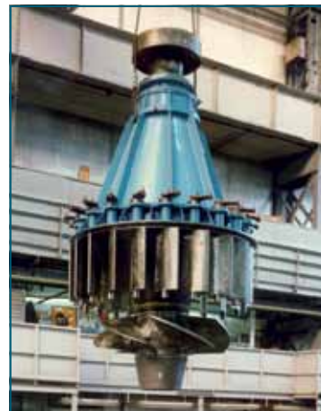
Fig. 3. The turbine upper cover with the guide vane assembly and the rotor is being lowered, Datong project China
